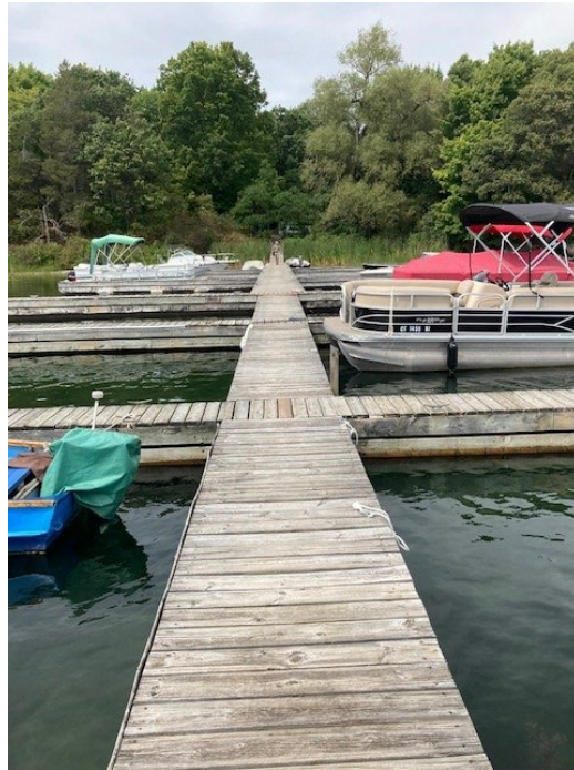
Photo 3 showing docks, shoreline, and access walkway
